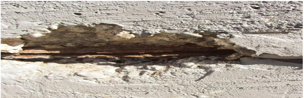
Fig 3 : Spalling due to rusting rebar.
