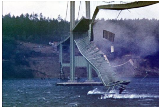
Figure 1: The collapse of Tacoma Narrows bridge on November 7, 1940 [6].
